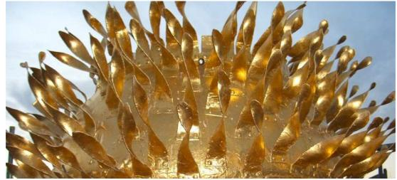
Hare & Humphreys Ltd carried out the re-gilding of the flaming orb, restoring its brilliant shine with the application of over 30,000 leaves of gold. Genuine 24 carat gold leaf was used in two layers, and applied in very exposed conditions by their expert gilders. It was part of  $\pounds 4.5$  million refurbishment project and the Monument re-opened in February 2009
